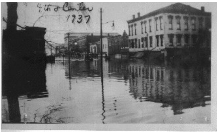
Fourth and Center Streets in Ironton during the 1937 flood.
